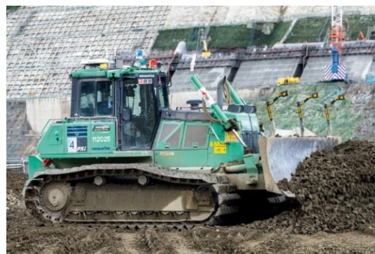
Naruse Dam Construction Project (Akita Prefecture)
