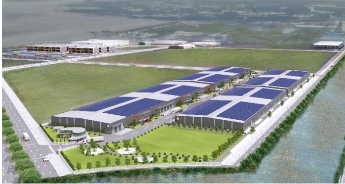
Core5 Hai-phong [distribution warehouse] (Vietnam)
